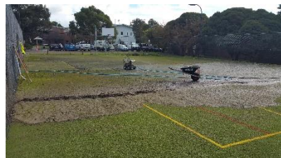
Before, after and during maintenance treatment
